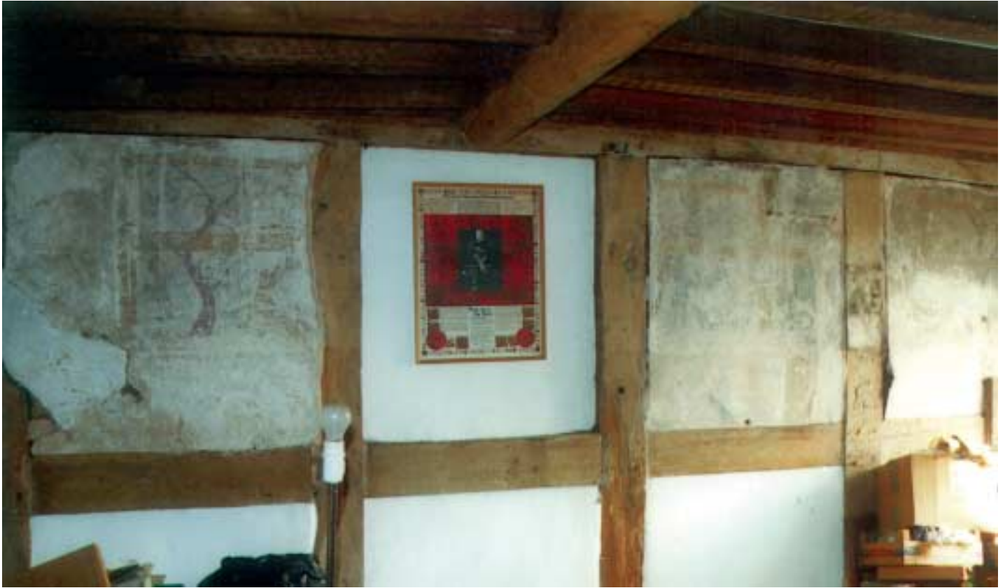
Figure 22 The drying-out process must be carefully controlled and monitored in order to protect historic decorations. Paintings on plaster, such as these early seventeenth-century examples in a Grade II*-listed house in Bewdley, are especially vulnerable to flood damage. (Robert Gowing)
