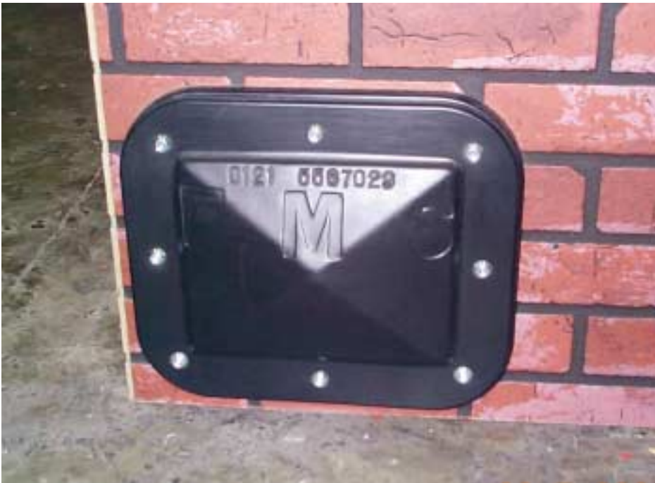
Figure 5 Airbricks can be sealed with temporary covers to keep out floodwater. (Courtesy of Flood Management Systems Ltd)
