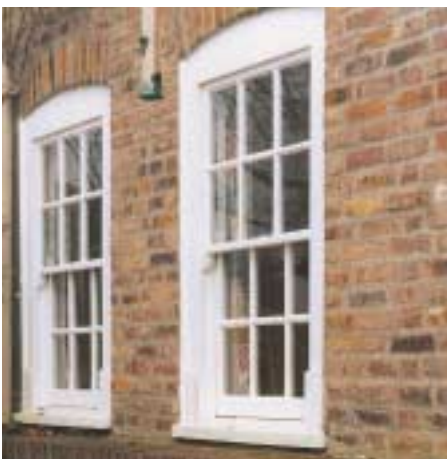
Figure 6 Sash window frames fitted with slots to hold temporary flood barriers. Painting the slots to match the frames helps them to blend discreetly into the background when not in use. (John Fidler)
