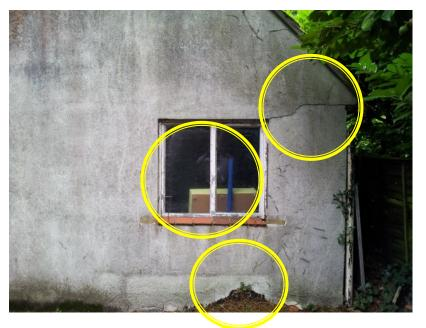
Summary of defects shown: Cracked render, timber decay and damaged render to lower wall.
