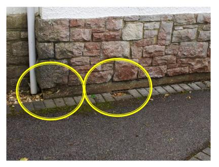
Summary of defects shown: A partially blocked sub-floor vent and some damaged render.
